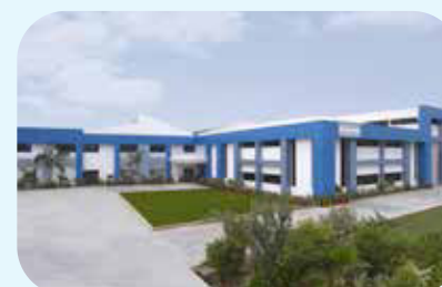
Harsha Engineers International Limited Moraiya Plant
