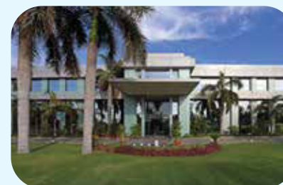
Harsha Engineers International Limited Changodar Plant
